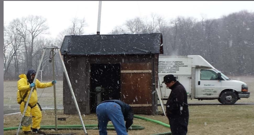
Replace Pump Station Before
