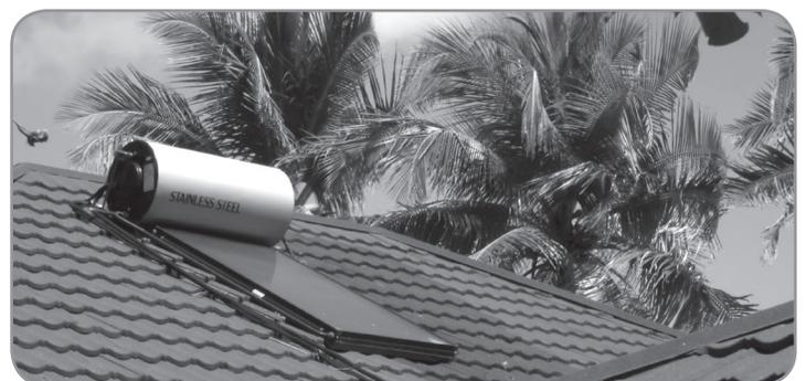
The heated fluid then goes to a storage tank where it heats water. The hot water may then be piped to a faucet or showerhead. Most solar water heaters that operate in winter use a heat transfer fluid, similar to antifreeze, that will not freeze when the weather turns cold.
